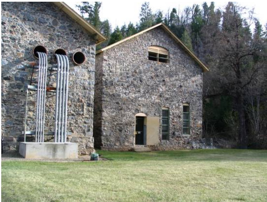
Photograph 1.1-1a Kilarc Powerhouse and Adjacent Land
