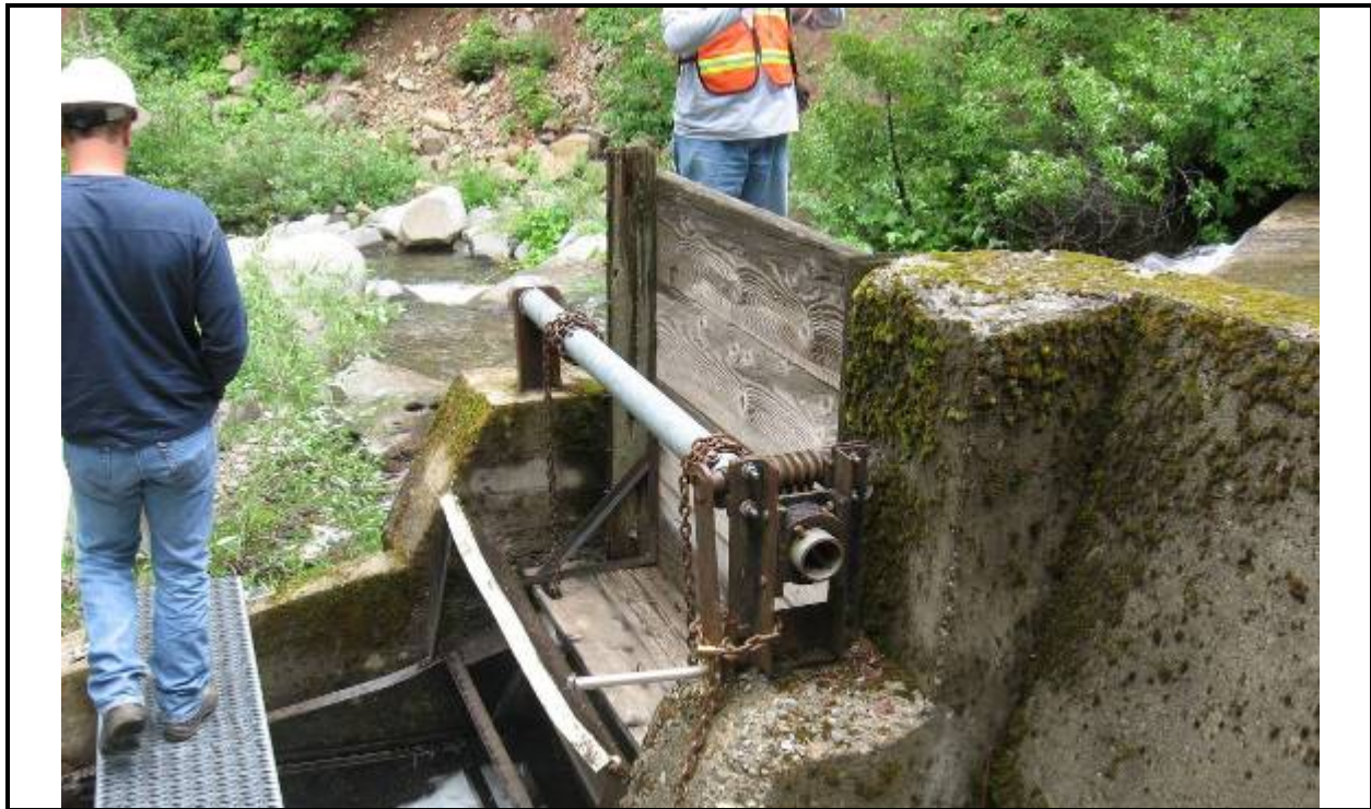
Photograph A-2. Kilarc Main Canal Intake.
