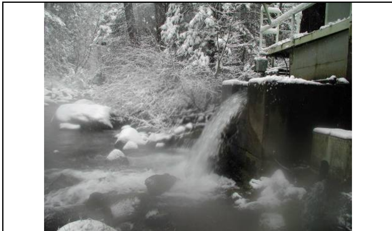
Photograph A-4. Flow Release at Kilarc Main Canal Diversion for Bypass Flows.
