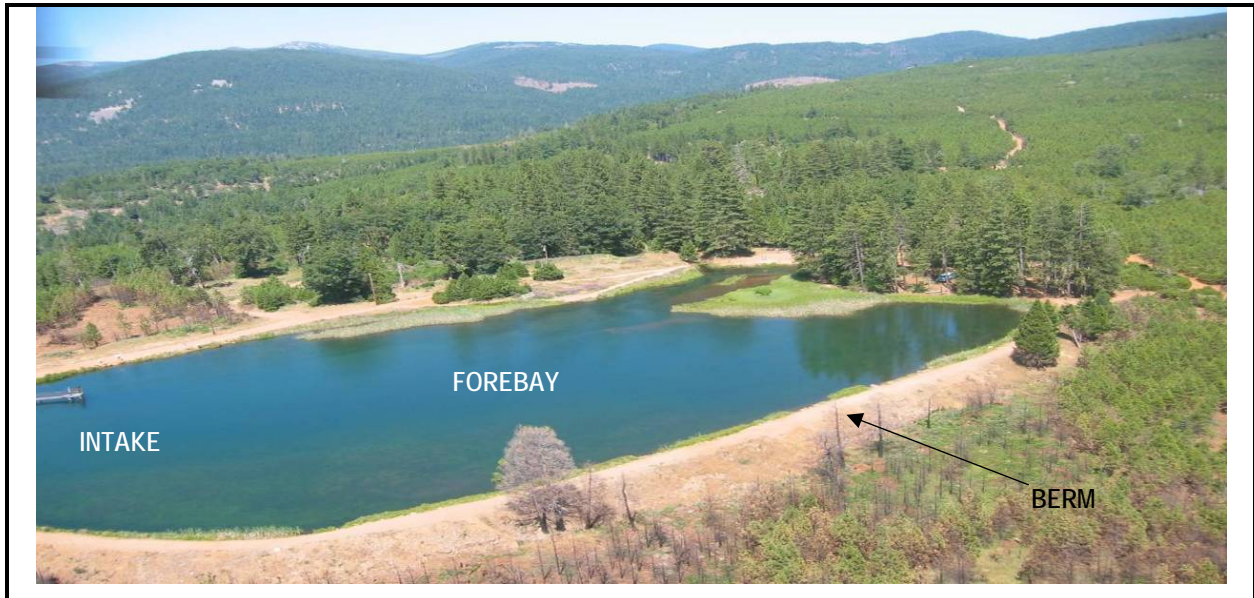
Photograph A-9. Kilarc Forebay Spill Channel.
